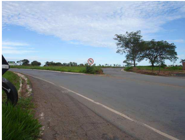
(a) Sentido BH-BSB
