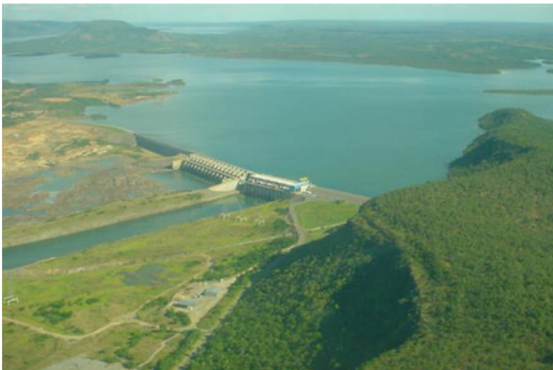
Figura 19: UHE Lajeado (INVESTCO, 2008)
