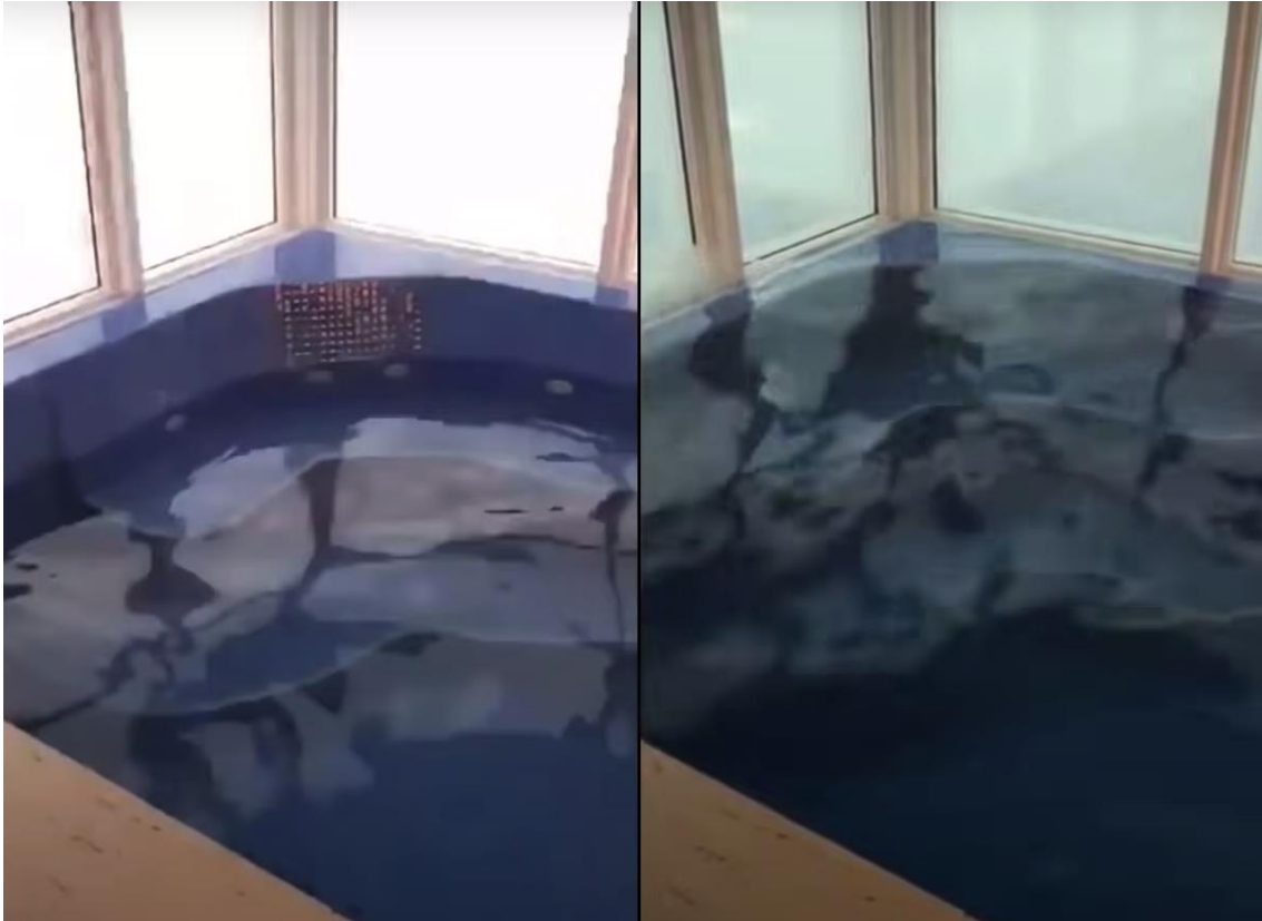
Figure 1-2 - Water displacement due to a building's oscillation during a storm (source: https://youtu.be/3YXrOFr4H9Q , accessed on January 16 2023)
