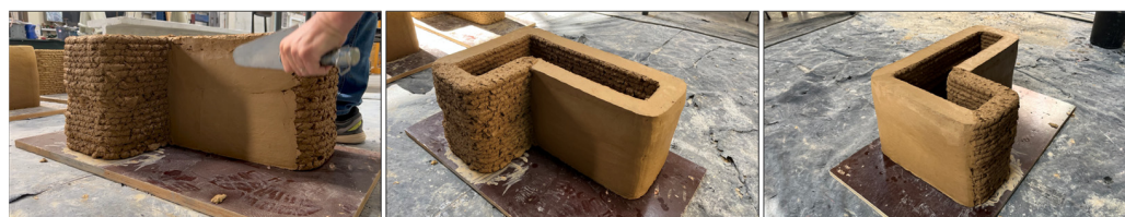
Figure 18. Surface-smoothing process for Kraftterra wall three days after printing.
