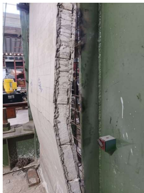
Figure 10. EPS visual inspection after failure of panel.
