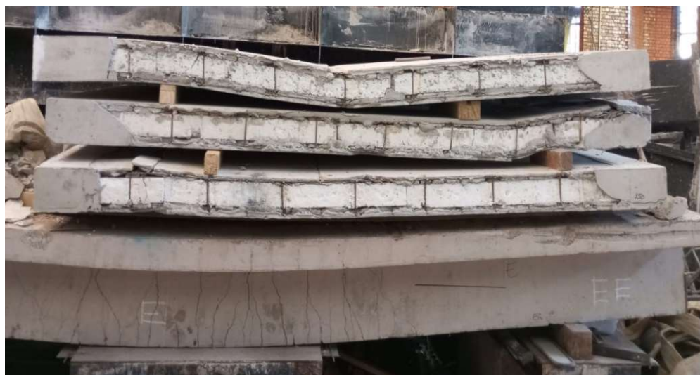
Figure 11. EPS visual inspection after failure of panel PA1, PA2, and PA3.
