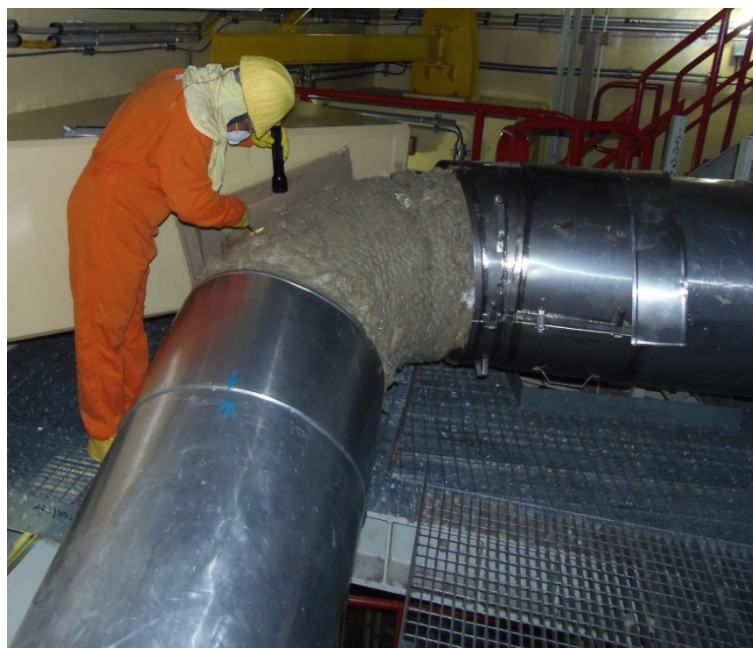
Figure 15: Inspection in main feedwater line and pipe whip restrain support
