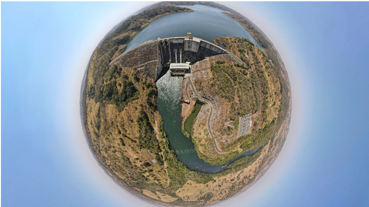
Figure 3.45 – Process image from the Hydroelectric Dam at São Marcos River
