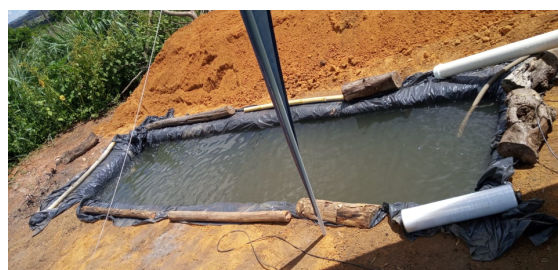
(b) Trench prepared for testing.
