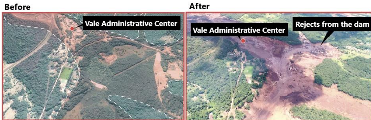
FIGURE 1 Feijão Dam in Brumadinho before and after de rupture ( Google Earth , 2019).
