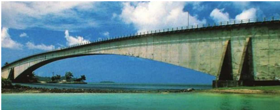
Figura 4.11: Ponte Koror-Babeldaob (Bažant et al. , 2010).
