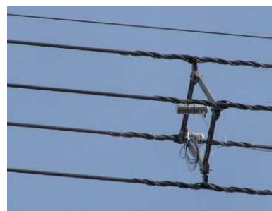
(c) Pavica 06P04 e Vibrec 500 instalados
