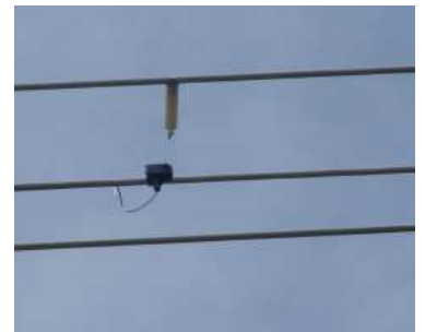
(c) Vibrec 500 instalado
