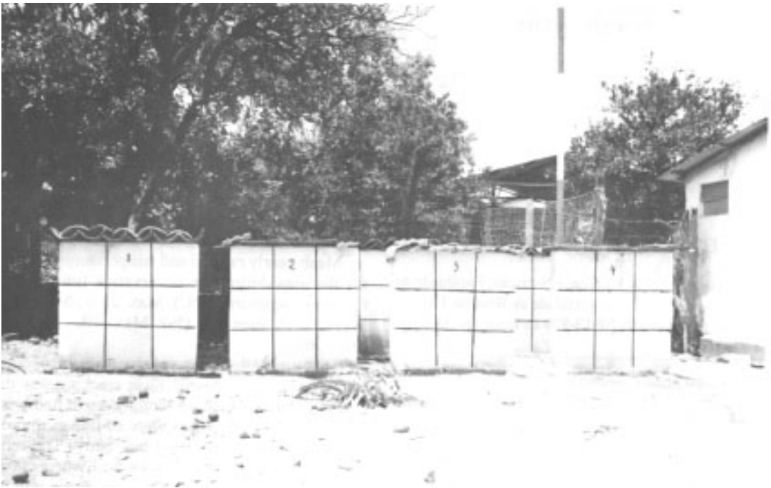
The six walls referred to in the text; two walls can be only glimpsed behind on the right.
