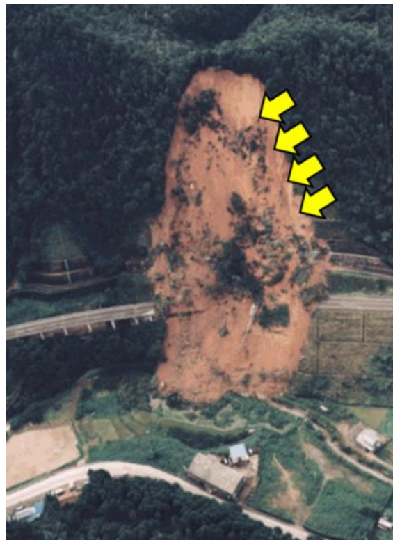
Fig. 6.5. Panoramic view of the Tokai-Hokuriku Expressway slope failure. Modified from Ye (2004). The thick yellow arrows indicate an observed zone of debris accumulation modelled in Fig. 6.4.
