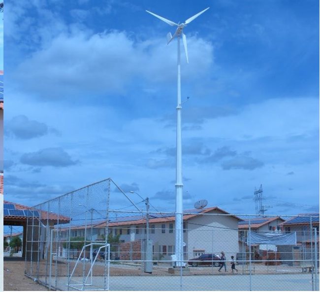
Figure 20. View of small wind tower installed in Juazeiro Source: C.A.G.Garcez Date: November 2013
