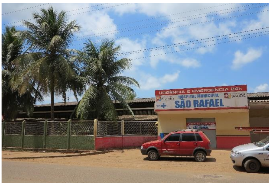
Figura 53 - Hospital Municipal São Rafael (Altamira, PA)
