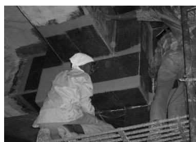
(b) Wadhwa Building, Mumbai - Índia
