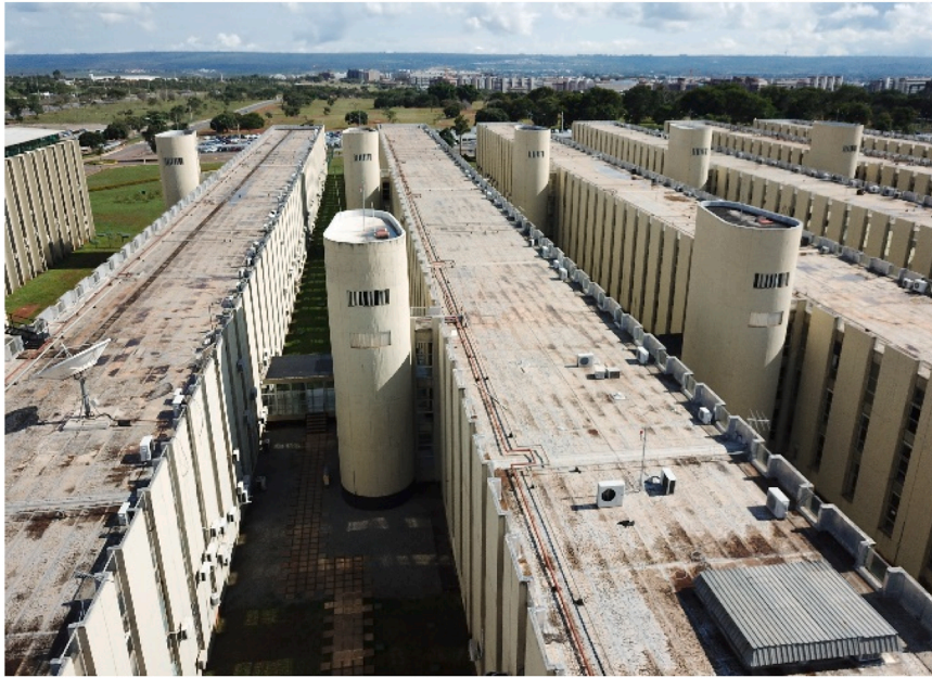
Fig. 2. Equipment arranged on flat roofs.
