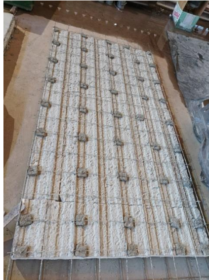
Figure 3. 13 - Placement of sleeves to keep mortar clear cover.
