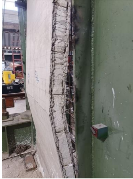
Figure 4. 15 - Side view of Panel PA1 after failure.
