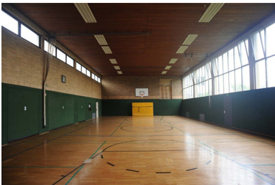
Fig. 6. Small gymnasium before renovation.
