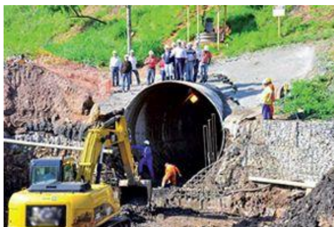
Figura 2.3 – Tunnel Liner , prefeitura de Rio Claro (SP) (Nakamura, 2012).
