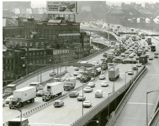
Figura 254 - Boston: Fitzgerald Expressway (1964).
